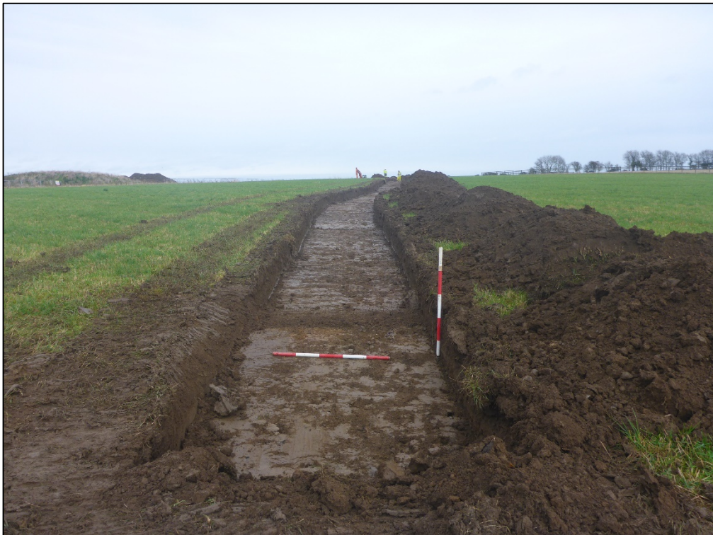
Plate 2 Test trench 5, looking northeast
